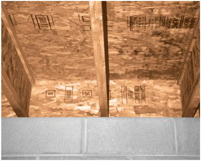
In this application, an engineered wood Rim Board is installed between the foundation sill plate and the floor under a wall section. The Rim Board matches the depth of the I-joists used in the floor framing.
